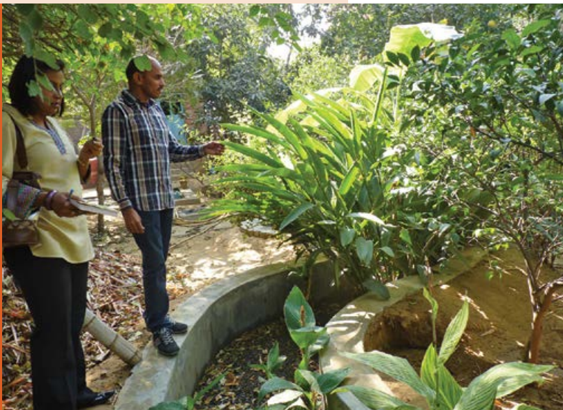
A project team inspects constructed wetlands in Ritu, Delhi, India, designed to filter out surface contaminants and silt that otherwise would discharge directly into nearby bodies of water. [Photo: RTI project staff]
