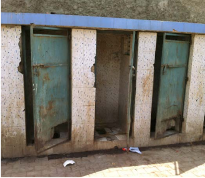
A public block toilet facility in a low-income area of Ahmedabad. Poor maintenance leads to open defecation around the facility.
