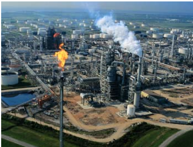
During the processing of oil and natural gas, methane leaks out from refinery equipment that is corroded or poorly installed. Directly inspecting the equipment with leak detection devices can help engineers identify and repair the worst leaks.
