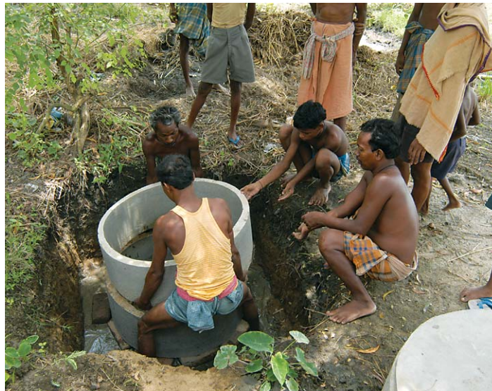
Members of a community in Orissa gather to build an individual household latrine.
